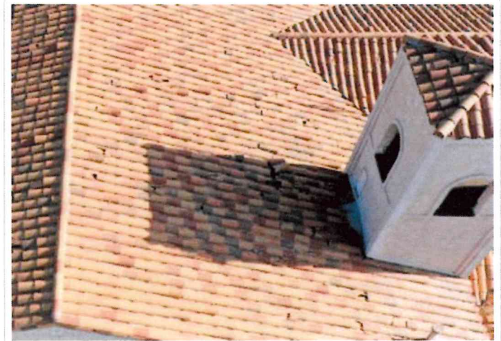
Roof overview: Roof areas surrounding the tower.
