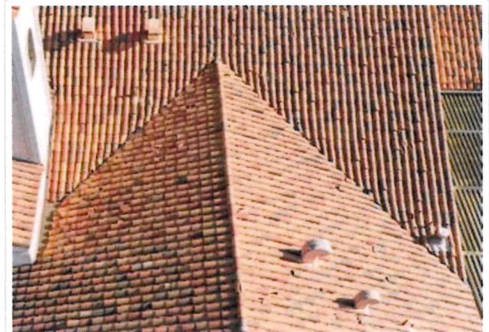
Roof overview: Multiple roof slopes and ridgelines.
