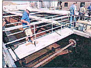
The Redlands Wastewater Treatment Plant is toured in 2018. The Redlands City Council and city staffers are backing increases to customers’ bills to pay for overdue upgrades at the plant.
