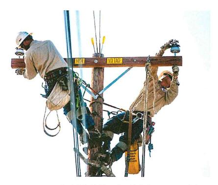
File photo by Watchara Phomicinda, The Press-Enterprise/SCNG Riverside Public Utilities workers Cory Schleiden, left, and Zach Neel climbed a 45foot pole to replace a transformer and a crossarm for voltage conversion project in Riverside in August.
