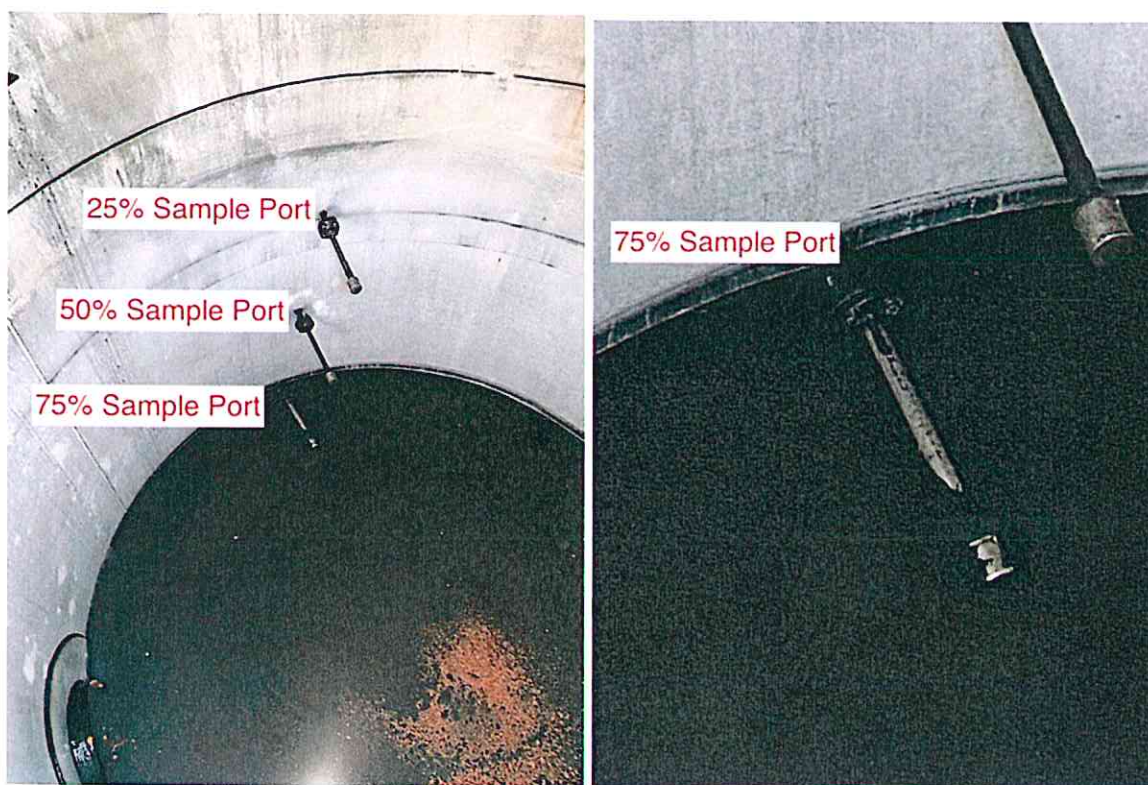
Figure 2 – May 19, 2022 photographs of Vessel 2 showing vessel is only filled to the 75% sample port (i.e., 25% of design capacity)
