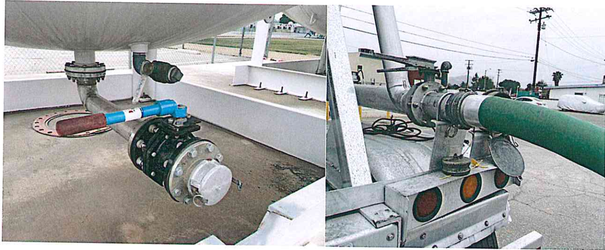
Figure 5 - Well 2. Left, 4" slurry-out port. Right, truck slurry connection
