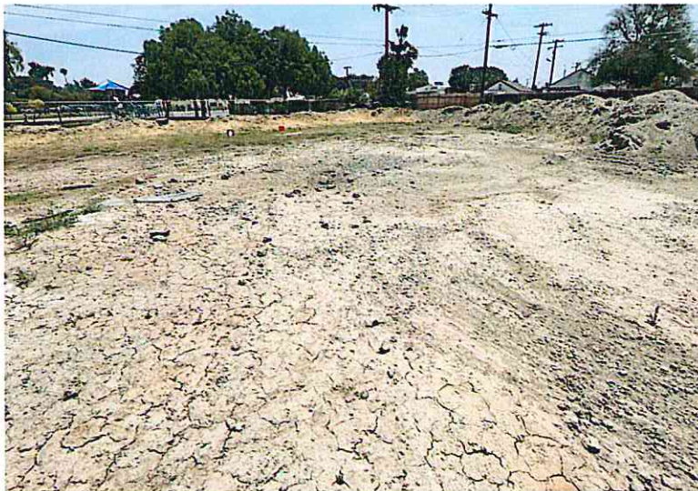
Figure 7 - Sedimentation Pond where backwash water is discharged. The missing GAC does not appear to be lost to sedimentation pond.
