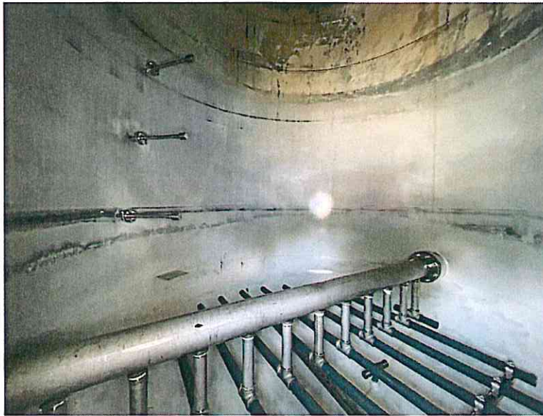
Figure 6 – Vessel 2 interior after pressure cleaning including manifold system and sample taps
