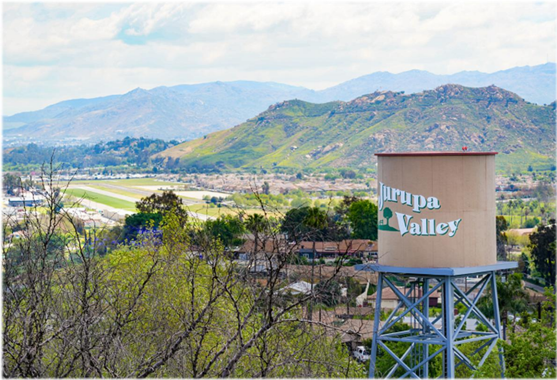
Figure 2.3: Cell Phone Tower Disguised as a Water Tower in the City of Jurupa Valley
