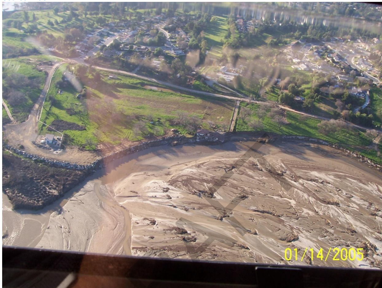
Photo B.2: Aerial Photo of Damage - January 14, 2005 Source: RCSD
